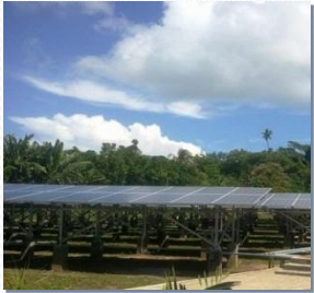
Bunaken 300 kW PV Plant, isolated grid
